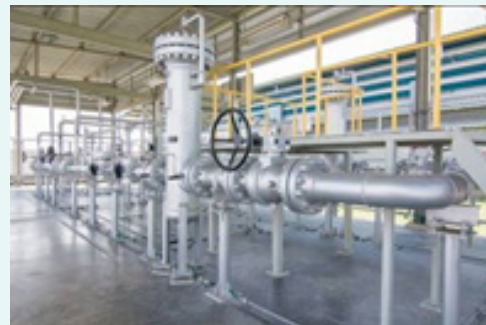
Metering system of natural gas quality improvement plants
