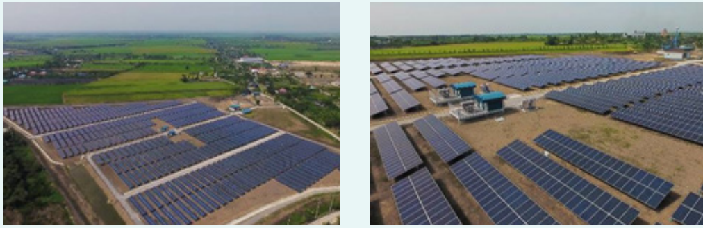
Solar power plant, Bangpasee Subdistrict, Bang Len District, Nakhon Pathom
